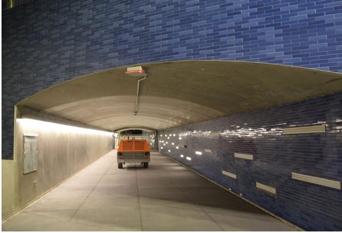
Photo 1 - Ped tunnel looking west
