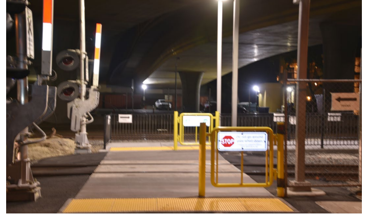
Photo 2 - Ped grade crossing
