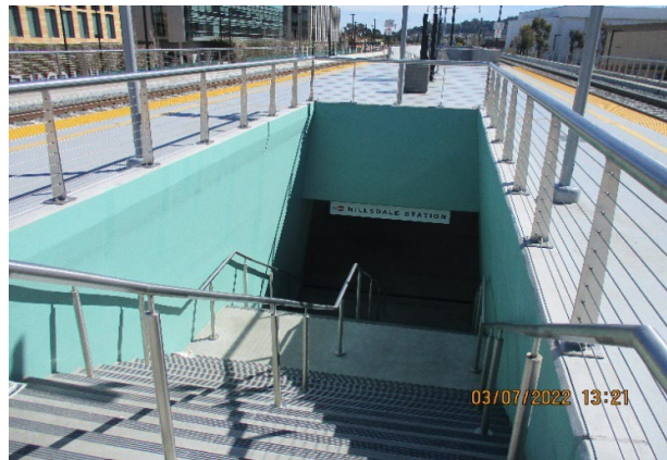
Photo 4 - Stairs Paint Touchup at Hillsdale Station
