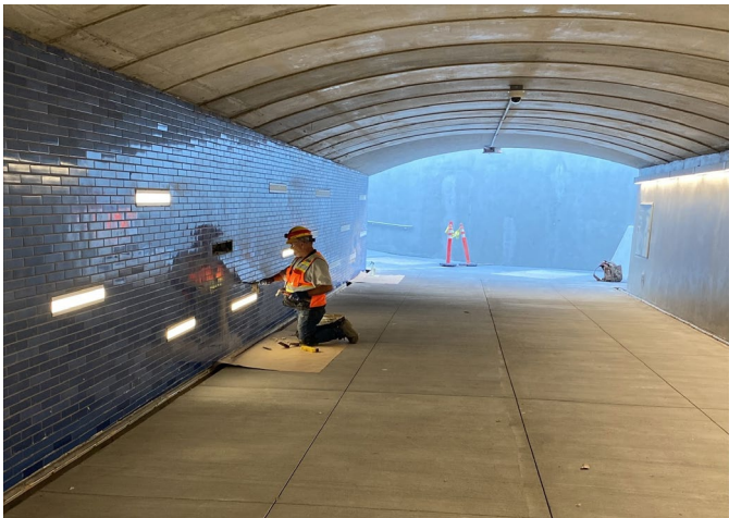
Photo 3 - Ped Underpass looking east
