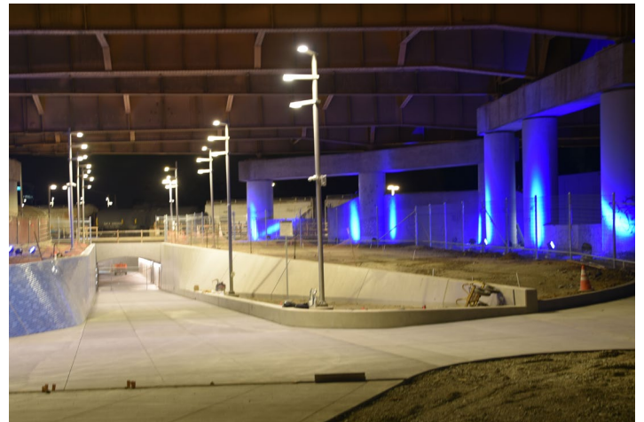
Photo 4 - Poletti Way looking towards East Plaza
