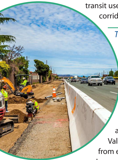
Photo: Construction along Highway 101
