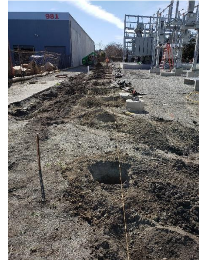
Excavating for site fence foundations at TPS-2.
