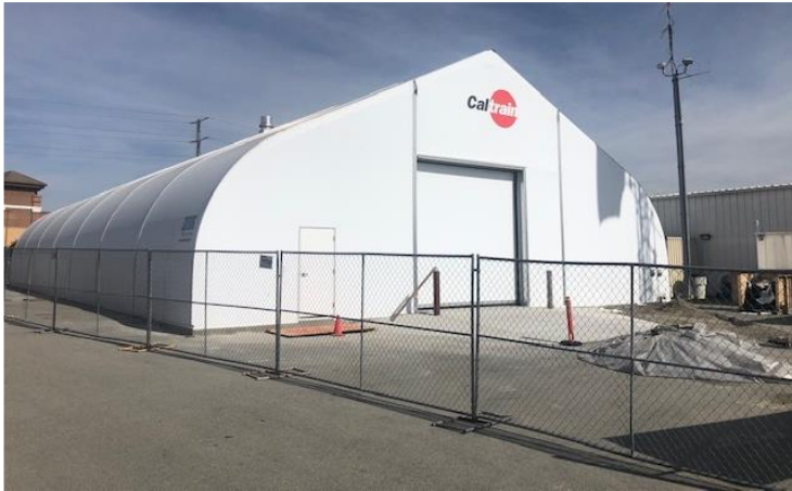
Parts Storage Warehouse
