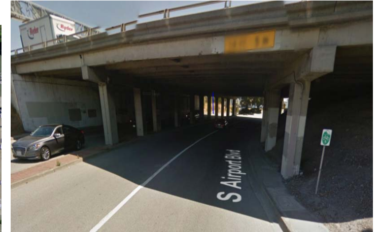
US 101/S. Airport Blvd Undercrossing
