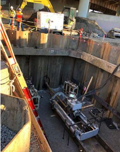
Shoring and Main installation - West Plaza
