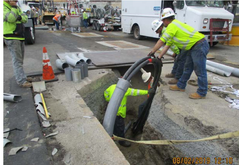
Routing from Splice box to termination point
