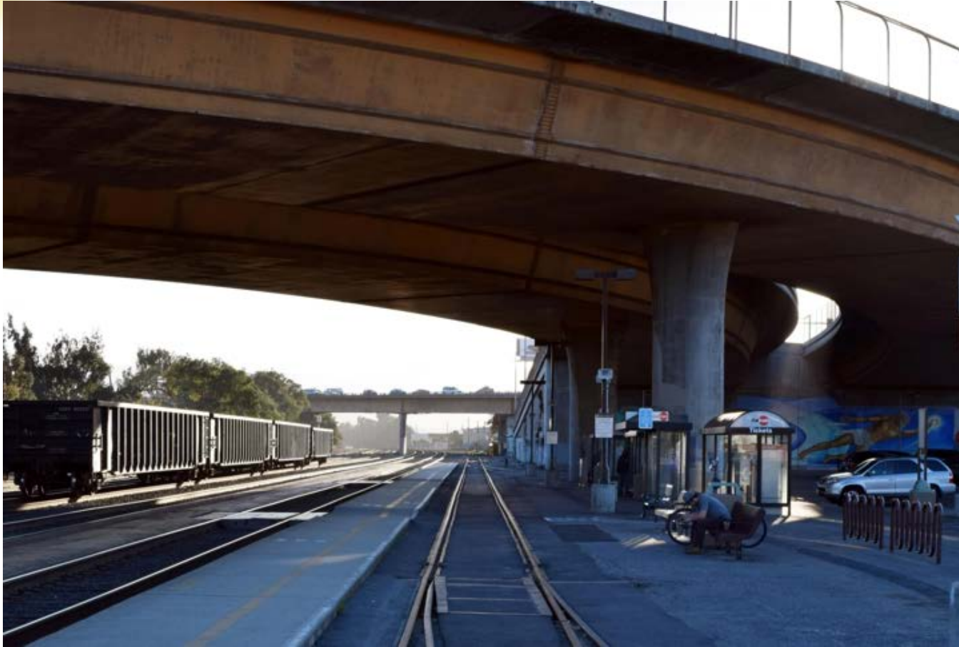
Existing Platform – South San Francisco Station Boarding
