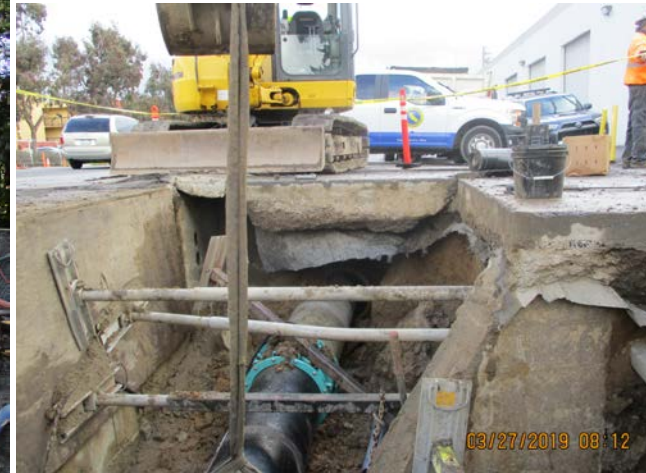
Water main tie in East Grand Ave.
