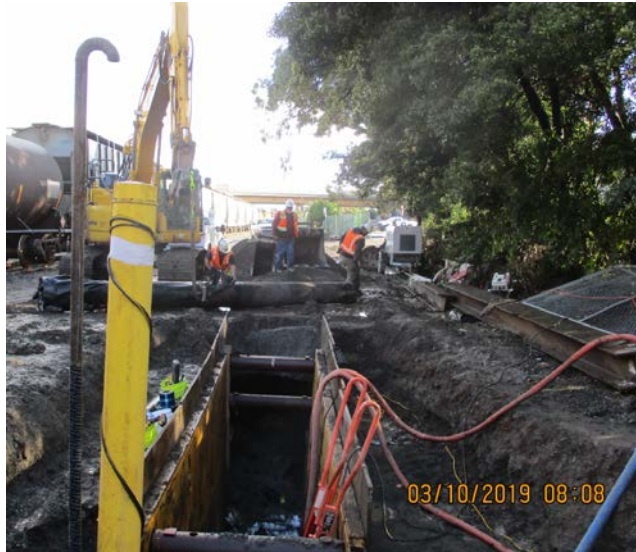
18 inch water main East side UPRR track
