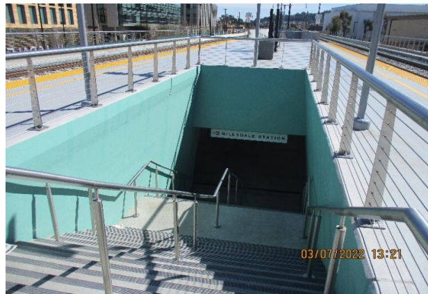
Photo 4 - Stairs Paint Touchup at Hillsdale Station
