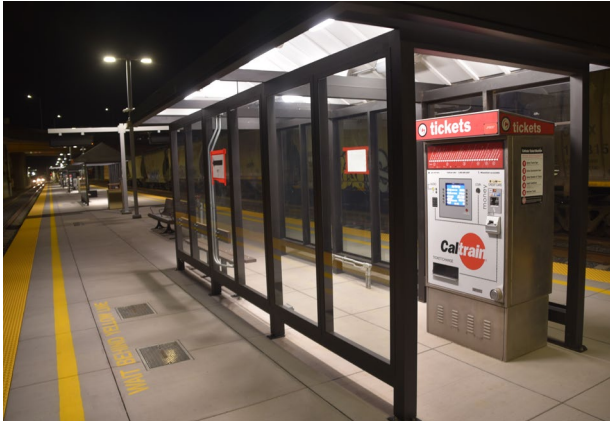
Photo 1 - Shelter with ticket machine
