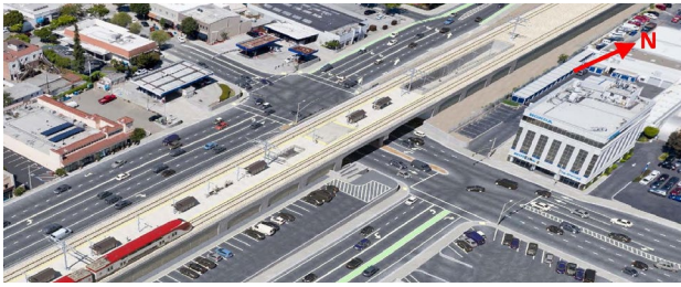
Photo 1 - After construction (rendering)
