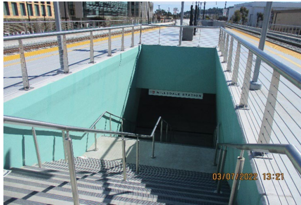
Photo 4 - Stairs Paint Touchup at Hillsdale Station
