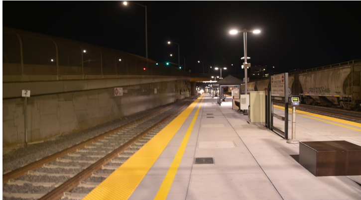
Photo 4 - New platform looking north MT-2
