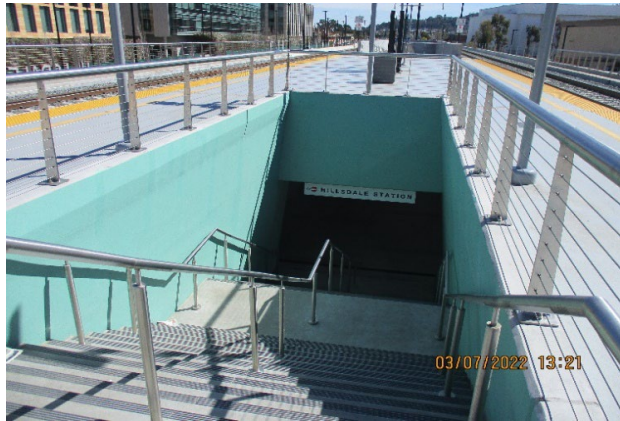
Photo 4 - Stairs Paint Touchup at Hillsdale Station
