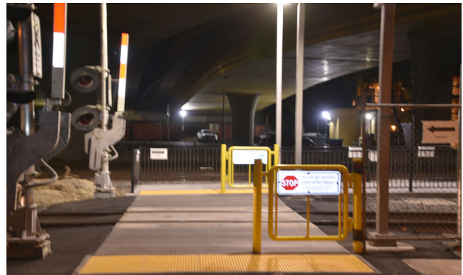
Photo 2 - Ped grade crossing
