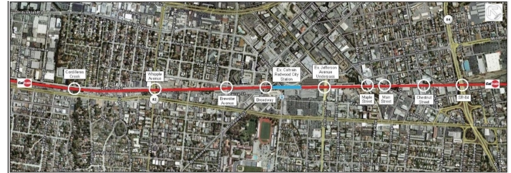
Source: BKF for San Mateo County Transportation Authority, "Grade Separation Program Footprint Study, City of Redwood City" (September 2009), p. 1
