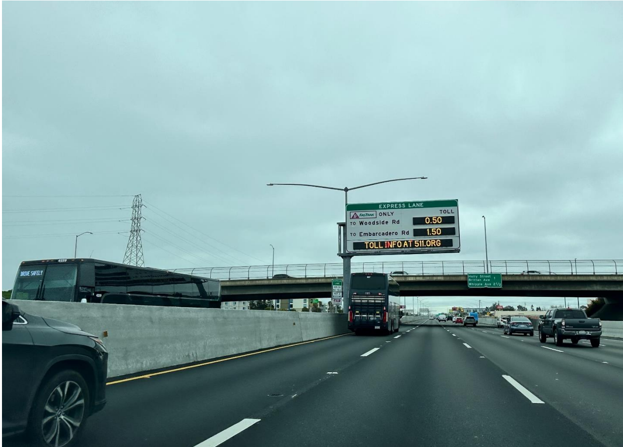
FULLY OPERATIONAL EXPRESS LANES
