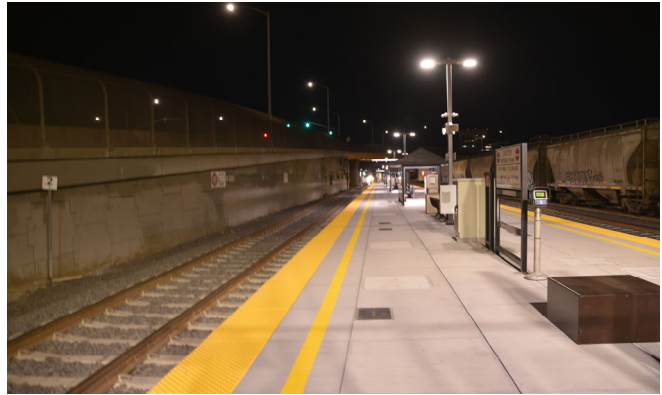
Photo 2 -New platform looking north MT-2
