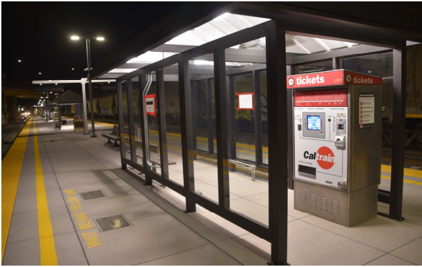
Photo 1 - Shelter with ticket machine
