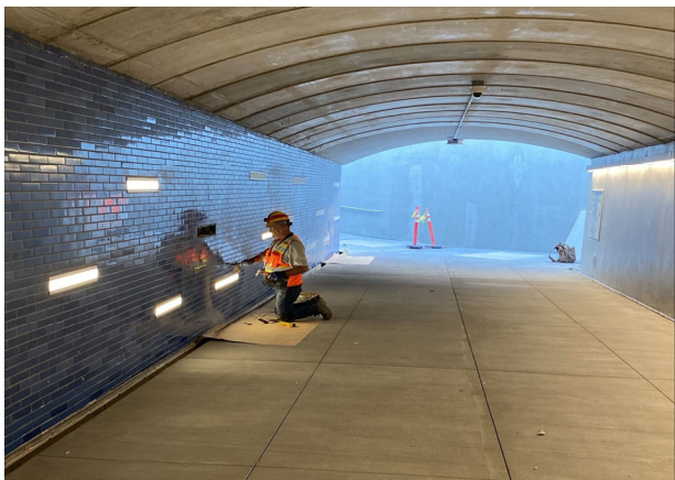
Photo 3 - Ped Underpass looking east
