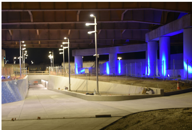
Photo 4 - Poletti Way looking towards East Plaza
