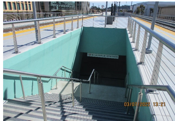
Photo 4 - Stairs Paint Touchup at Hillsdale Station
