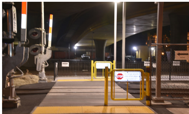
Photo 2 - Ped grade crossing
