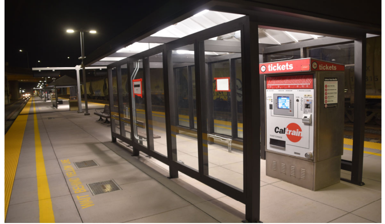
Photo 2 - Shelter with ticket machine
