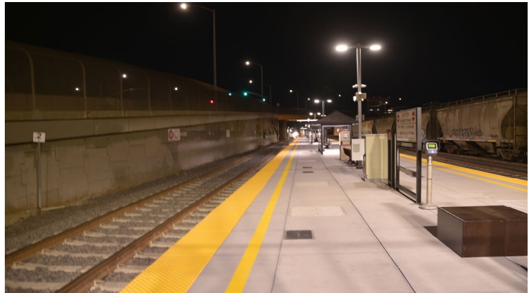
Photo 4 - New platform looking north MT-2
