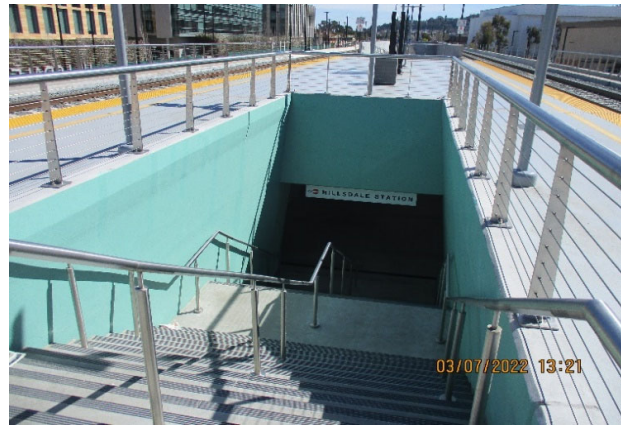
Photo 4 - Stairs Paint Touchup at Hillsdale Station
