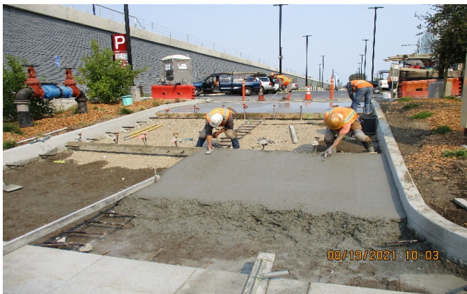
Photo 3 - New Driveway for Bike Path
