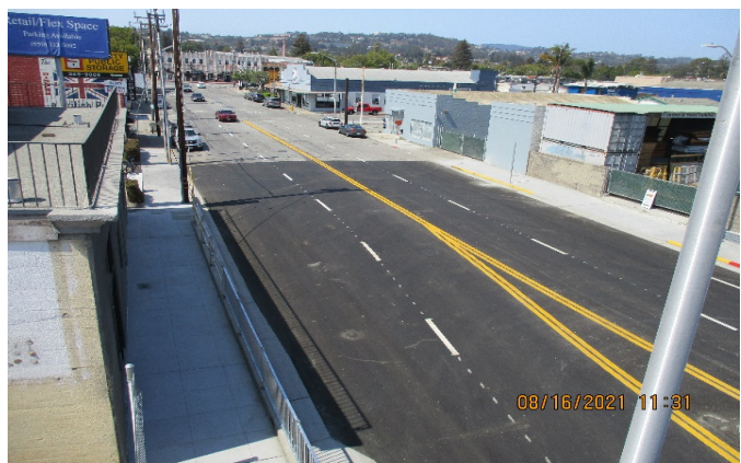
Photo 4 - 25th Ave. Opening
