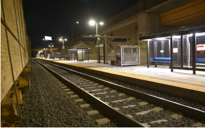
Photo 1 - New platform looking south
