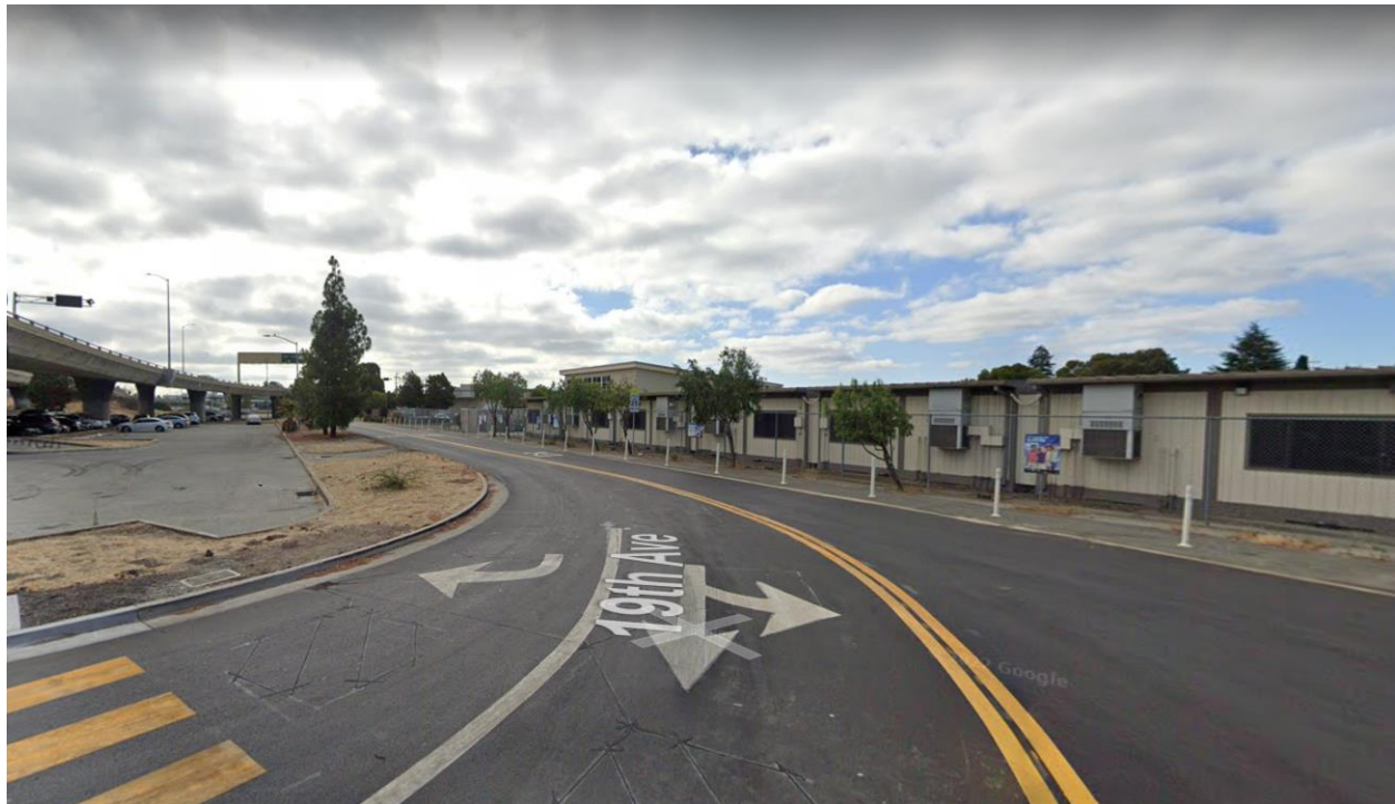
Figure 2-13: Park and Ride lot (left) and Fiesta Gardens International School (right) (Google Street View)
