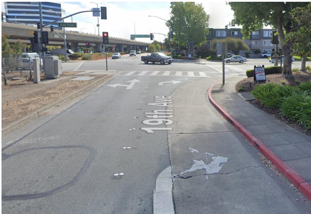
Figure 2-22: 19 th Ave. and Grant St. intersection (Google Street View)
