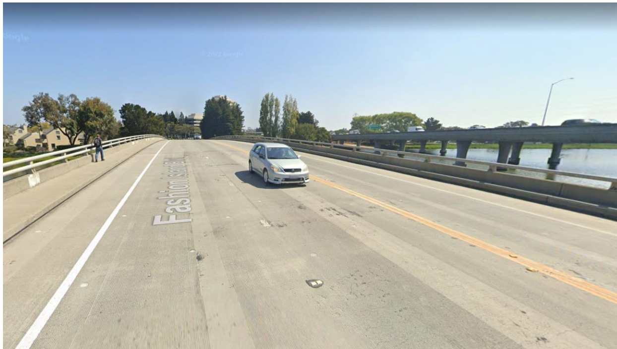
Figure 2-29: Fashion Island Blvd. over Seal Slough (Google Street View)
